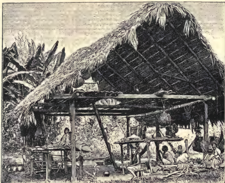
FIG. 170—A House in Central America
